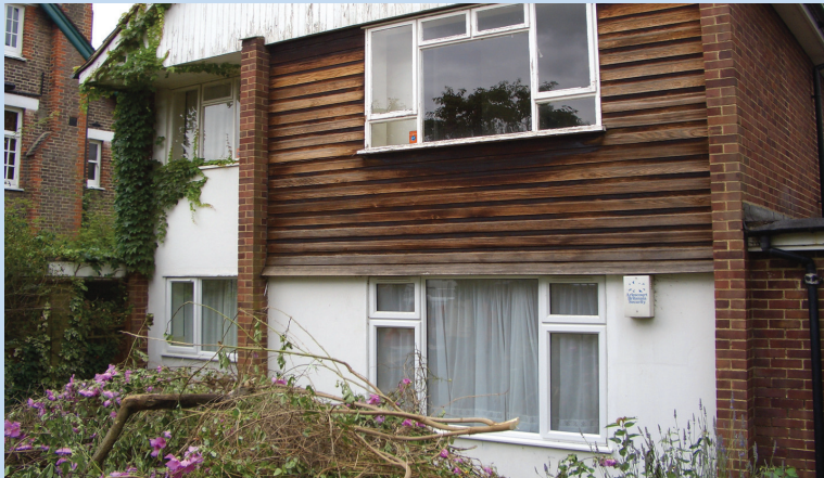
Project one before demolition
